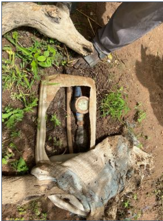
Figure 8: Water meters in Keur Malick Ndiaye. These meters are inside every Forest Garden and measured participants' monthly water use.
