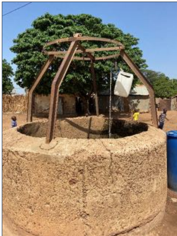
Figure 6: One of two community wells in Keur Birmane Ndoupi. Each haul brings up half a jerry-can of water (since the jerry-can is cut out in the middle for pouring), necessitating at least 40 haul to fill 20 jerry-cans of water for a single irrigation session.
